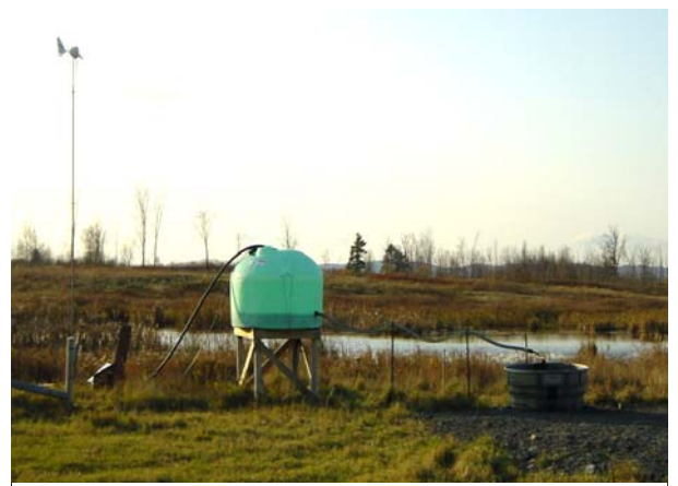
Figure 7: Stationary Solar-Powered and Wind Powered watering site
