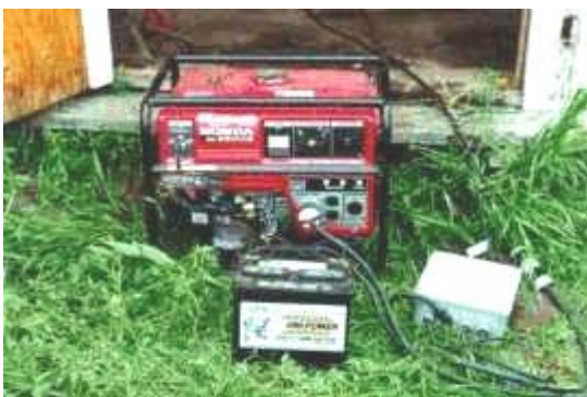
Figure 4: Gas-powered electric generator used to run an electric water pump.
