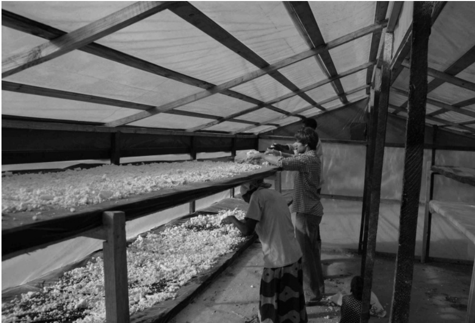
Figure 2: Inside the existing drying shed
