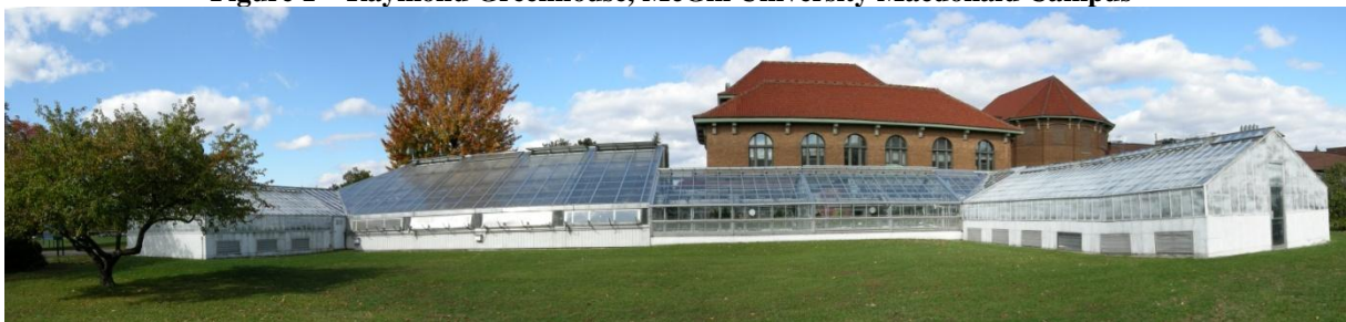
Figure 1 – Raymond Greenhouse, McGill University Macdonald Campus
