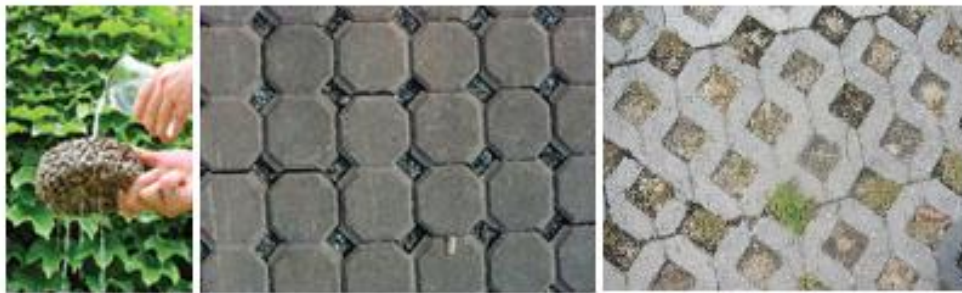
Figure 6. (a) Permeable concrete; (b) Interlocking concrete paving; (c) Grid paving
