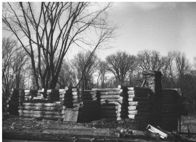
Chalet Pruche was built in 1947 by Macdonald College staff led by Layton Burnett. Hemlock logs from the forest were used to erect the building on top of the foundation of a former sugar house.
