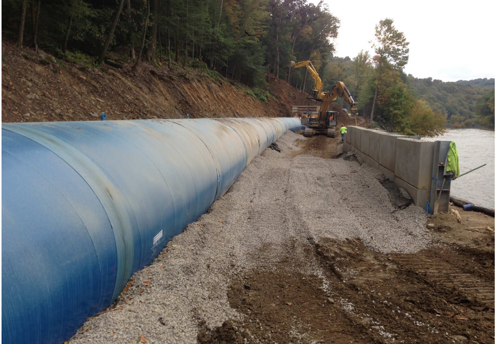
By the end of September there were 15 pieces of penstock pipe installed.
