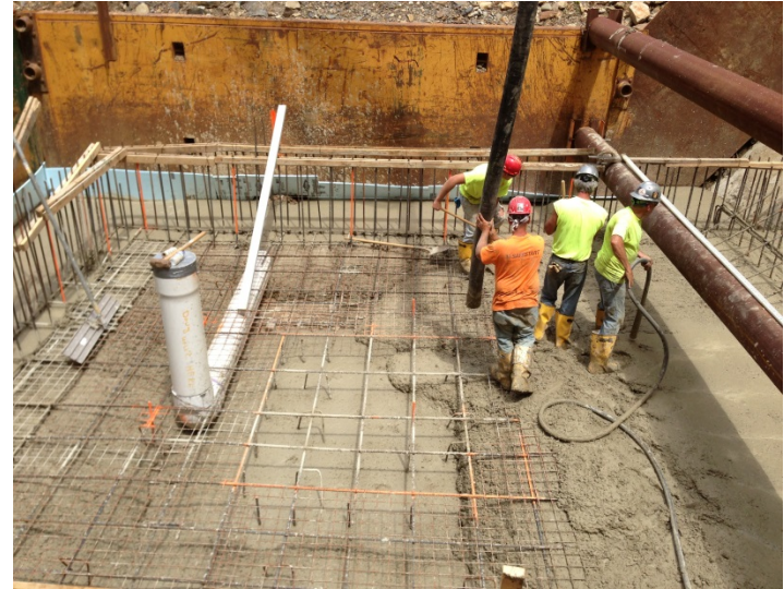
Pouring Valve Vault Base Slab
