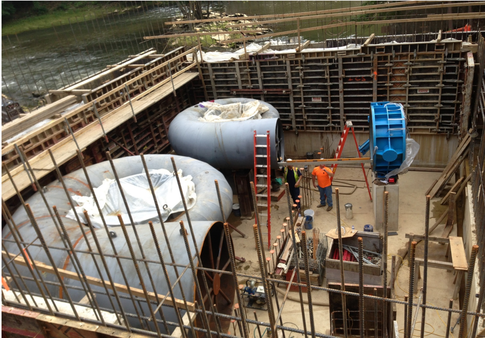
Spiral cases welded to conical draft tube. Small Turbine Shutoff Valve installed on concrete support.
