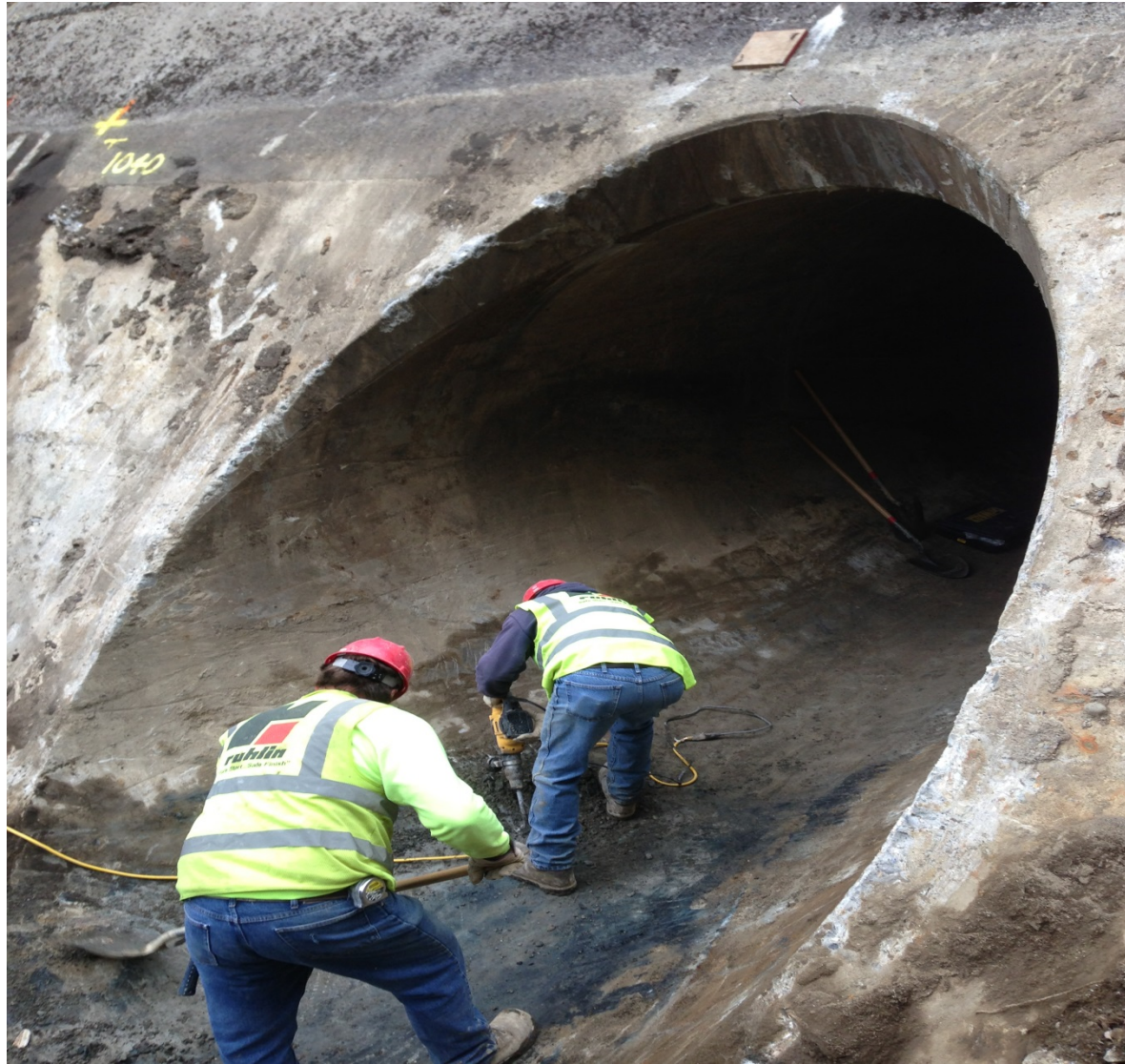
Uncovering the conduit in Monolith 15 on the downstream face of the dam.
