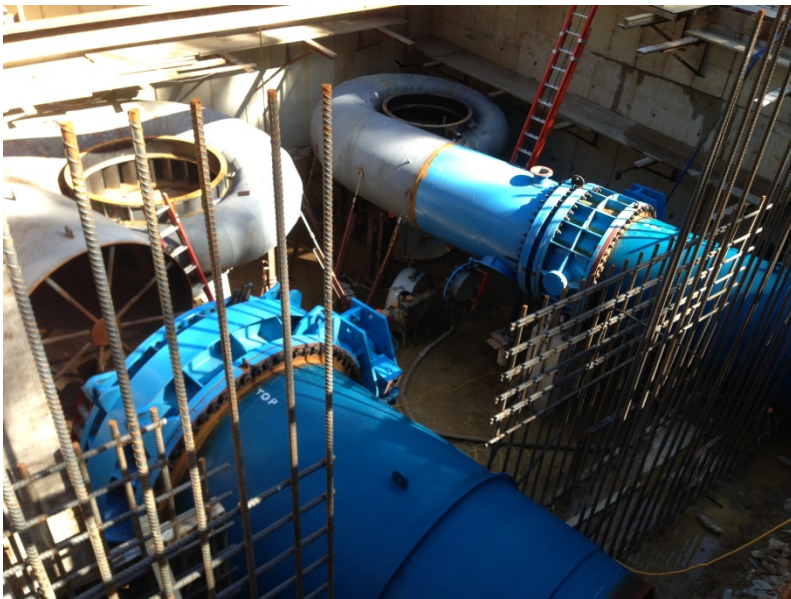
Installation of both spiral cases and TSV's in powerhouse
