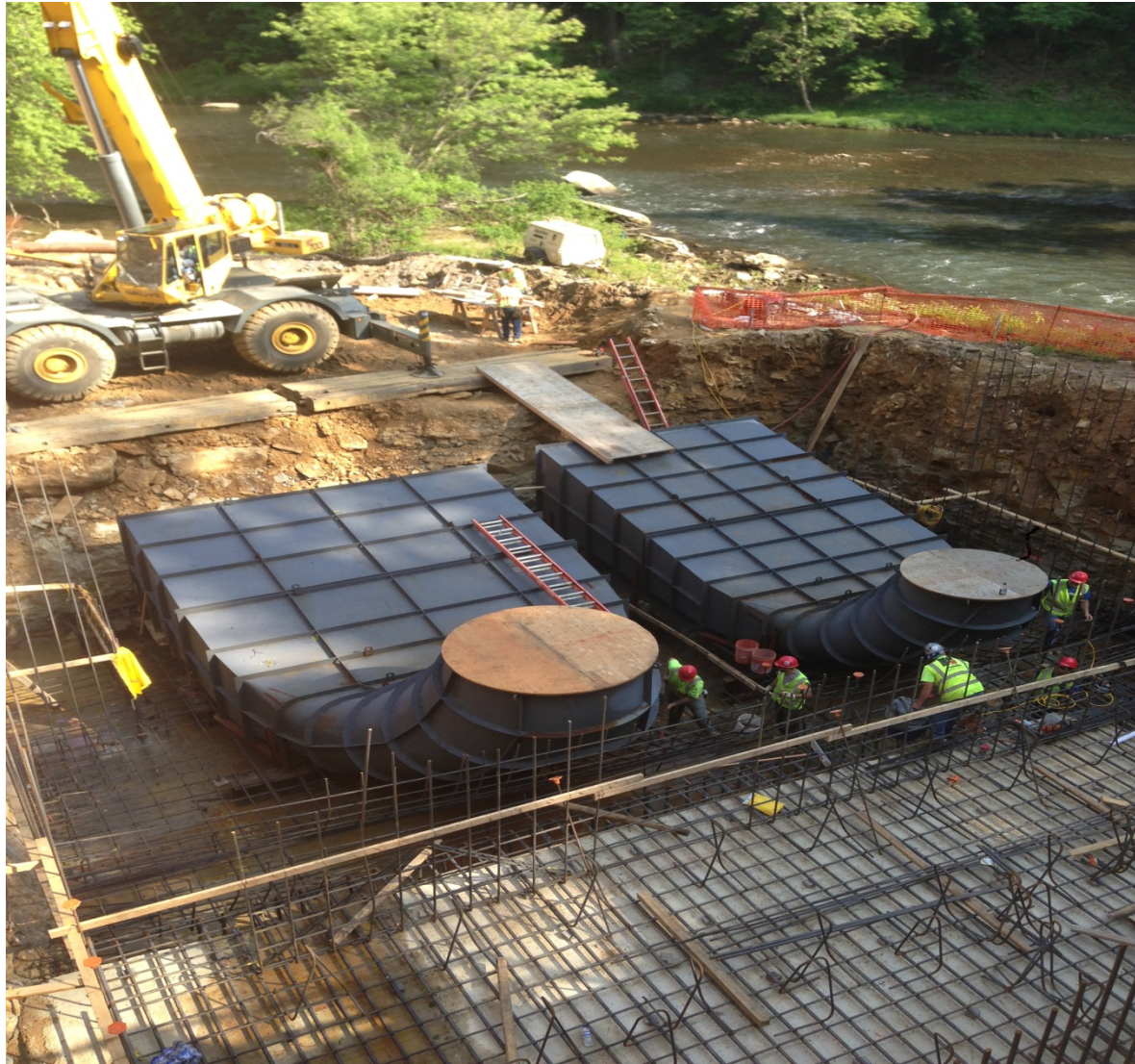
Draft tubes (Discharge) set in place in powerhouse end of May
